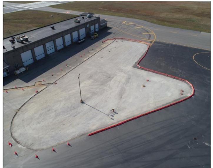
Photo shows excavated PFAS impacted soils removed and ready for asphalt cap as a permanent solution for mitigation.
