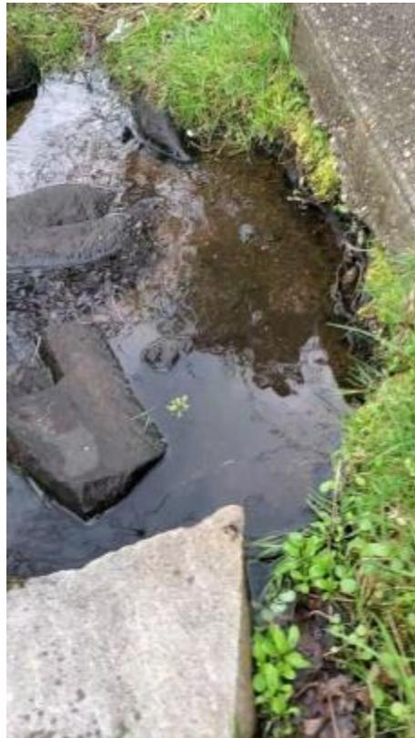
Water flow from pond under the sidewalk caused undermining.
