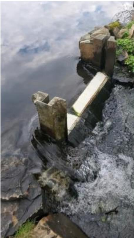
Stone damage and missing stones around the water control structure.
